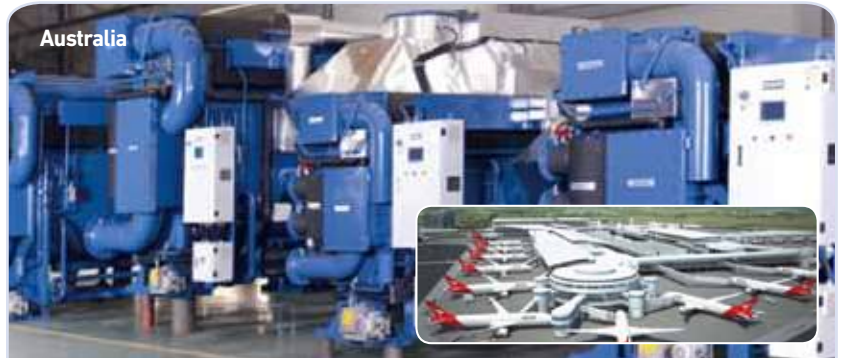
Qantas Trigeration at Sydney Airport CHP & HWR-L 3,642usRT(12,805kW)
