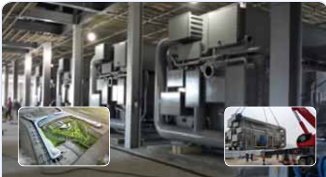
Incheon Interational Airport 2AB 8 sets 8,000usRT(28,128kW)
