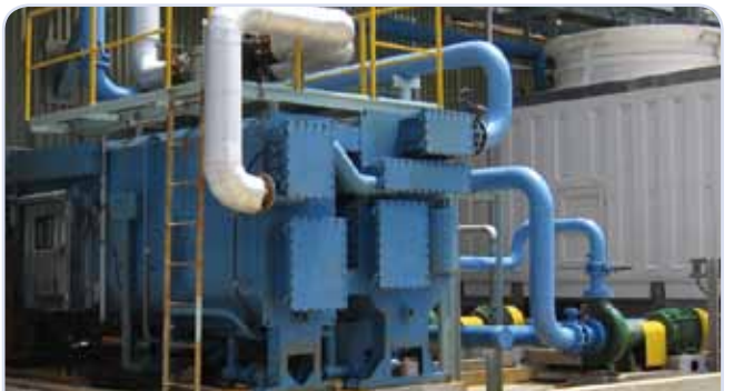
Youngpoong Seokpo Refinery 2AA 240usRT(844kW)
