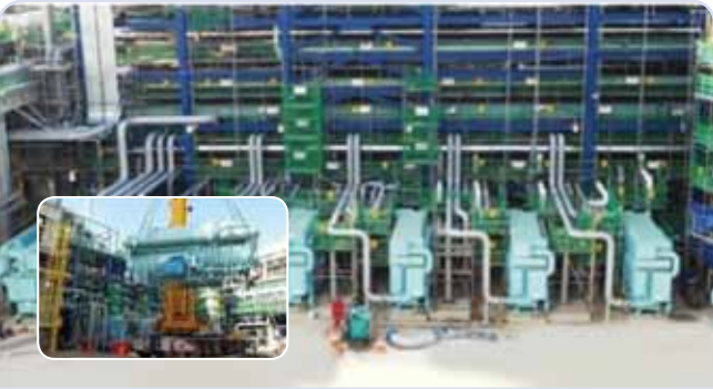
Samsung Total SW & HWAR-L 9,787usRT(34,411kW)
