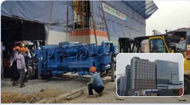
Hwaeom Building Munjeong-dong 2AB 270usRT(949kW)
