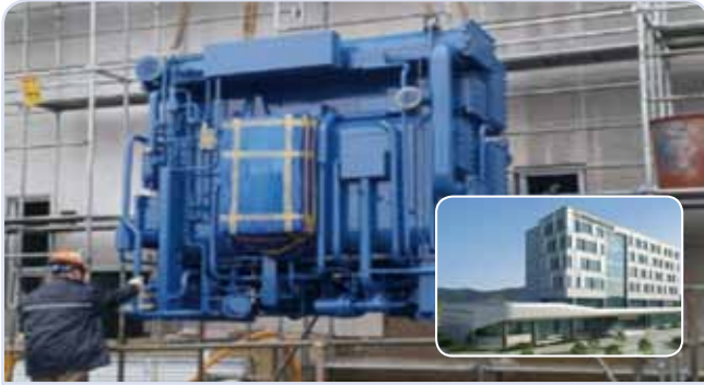
Korea Elevator Safety Agency 2AB 150usRT(527kW)
